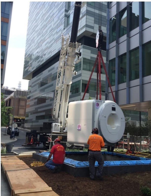
Trade partners hoisting the 7T MRI into the precast opening
